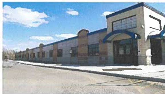
JOHN F. KENNEDY ELEMENTARY SCHOOL
